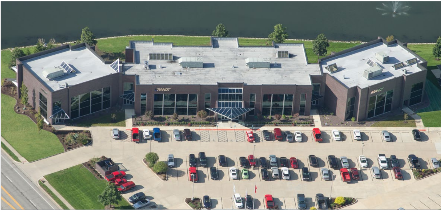
BRANDT Headquarters, Springfield, Illinois.
