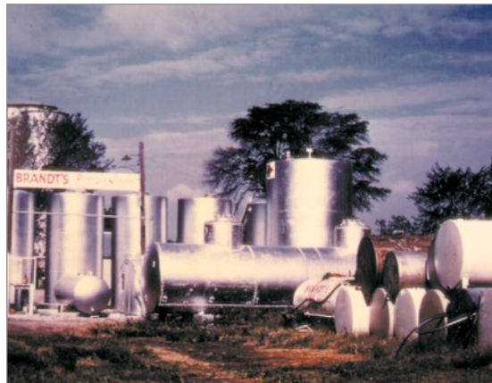
BRANDT's first plant in Pleasant Plains, 1957.
