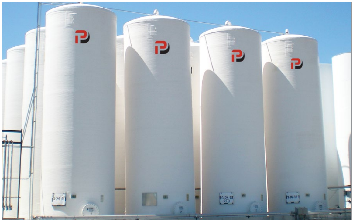
The Precision Tank company in Virginia, Illinois, was formed in 1965.
